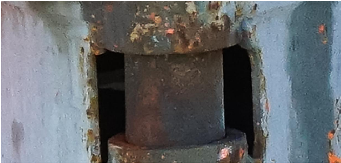
FLARE BOOM SUPPORT PIN DETAILS
